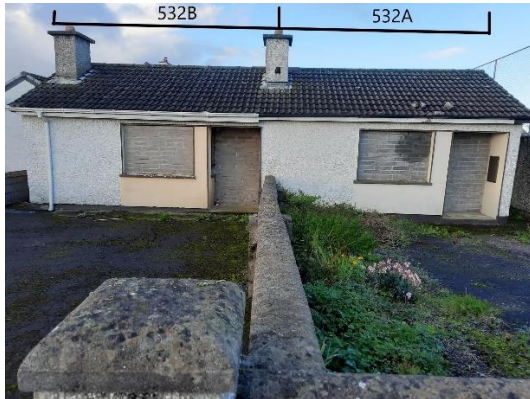
Pic 1: Units 532a and 532B.
